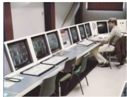
Fig. 3. Damatic control room.
