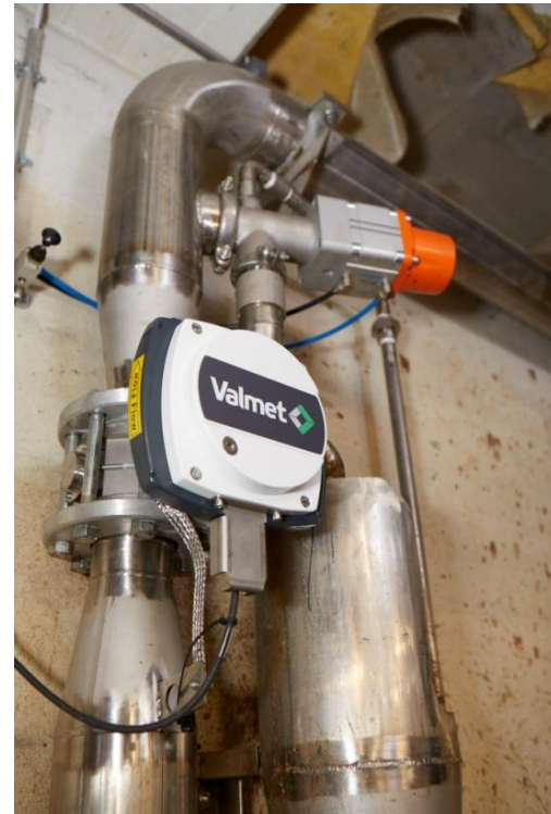
Fig. 4. Valmet TS microwave total solids transmitter
